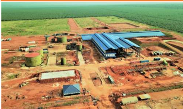
CONSTRUCTION OF OUR FIRST 30T/HR OIL MILL AT EXTENSION 2
