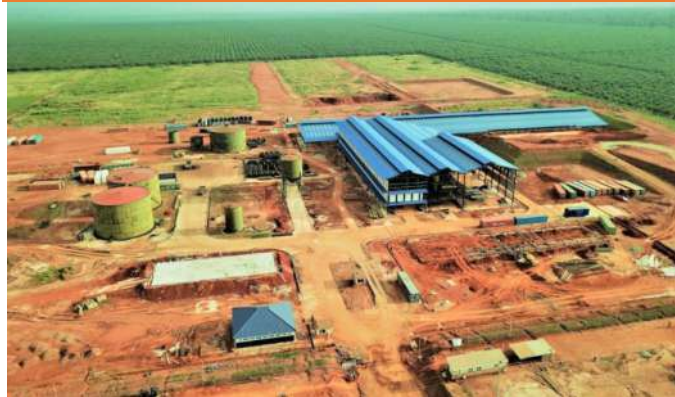
CONSTRUCTION OF OUR FIRST 30T/HR OIL MILL AT EXTENSION 2 IN 2020
