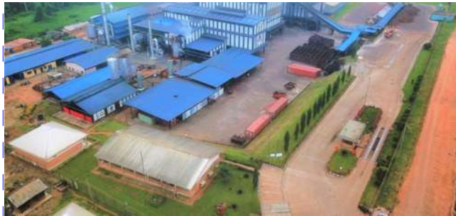
AERIAL VIEW OF THE 65T/HR OIL MILL AT THE MAIN ESTATE
