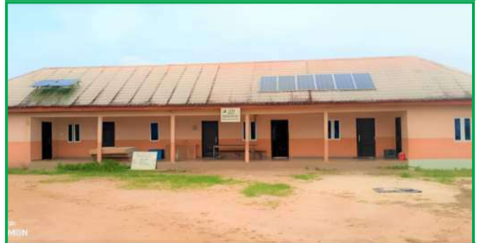
RENOVATED MATERNITY HOME AT OFUNAMA COMMUNITY
