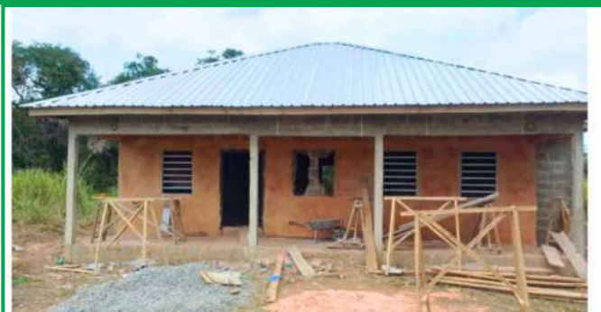
FIRST PHASE OF THE NIGERIAN POLICE POST AT SAFAROGBO COMMUNITY
