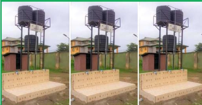
SEMI-INDUSTRIAL BOREHOLE AT INIKOROGHA COMMUNITY
