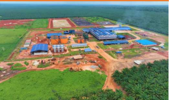
AERIAL VIEW OF THE COMPLETE 60T/HR OIL MILL AND PLANTATION OFFICE AT EXTENSION 2 IN 2023
