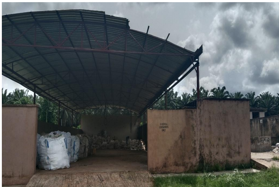
Plate 12: Empty Agrochemical Containers' Storage Compartment Covered with Aluminium Roofing Sheet to Prevent run-off during Rainfall
