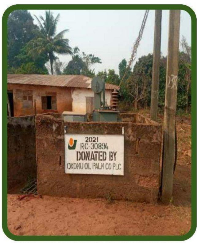
INSTALLATION OF 200KVA (33KVA/415) STEP DOWN TRASFORMER AT IRHUE COMMUNITY - 2021
