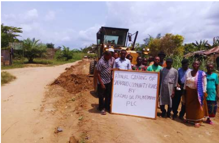
Road Grading In Progress
