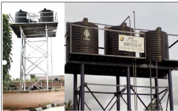
SEMI-INDUSTRIAL BOREHOLE AT THE PALACE OF THE IYASE OF UDO, OVIA SOUTH WEST LOCAL GOVERNMENT AREA & SEMI-INDUSTRIAL BOREHOLE AT MARIOGHIONBA (AT&P) COMMUNITY, OVIA SOUTH WEST LGA CONSTRUCTED BY OOPC
