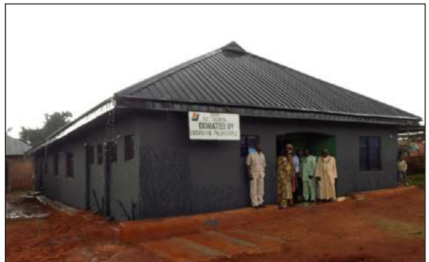
COMMUNITY TOWNHALL AT UMOKPE, UHUNMWONDE LGA, CONSTRUCTED BY OOPC
