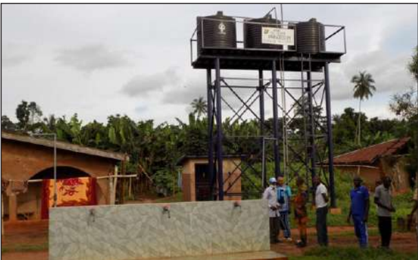
INDUSTRIAL BOREHOLE AT EKPAN COMMUNITY, UHUNMWONDE LGA, BUILT BY OOPC
