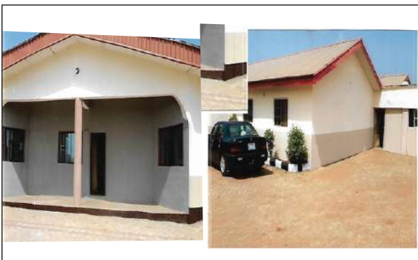
PALACE OF IYASE OF UDO, OVIA SOUTH WEST LGA, RENOVATED BY OOPC
