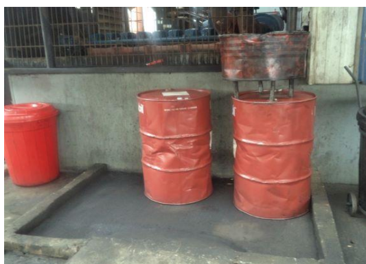
Plate 3.5: Bund Wall around Hazardous Chemicals
