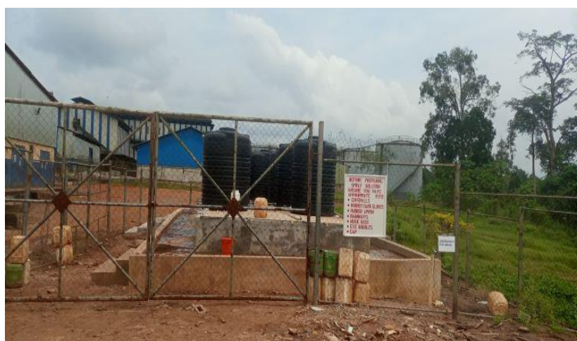
Plate 3.6: Bund Wall around Pesticide Mixing Tank at Agric Office
