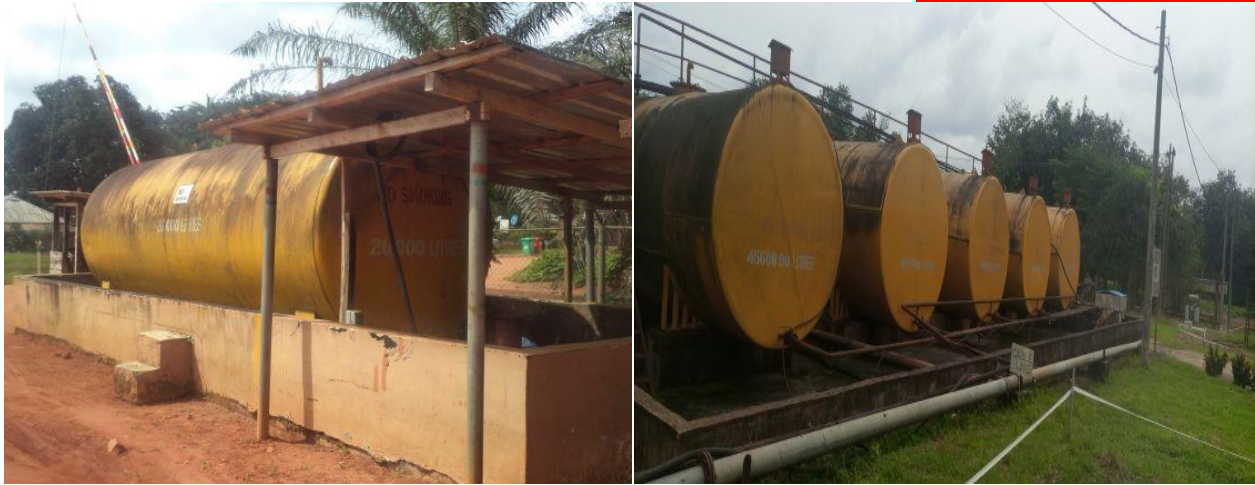
Plate 3.9: Provision of Bund Wall against Spillage at Main estate Filling Station and Rubber Factory
