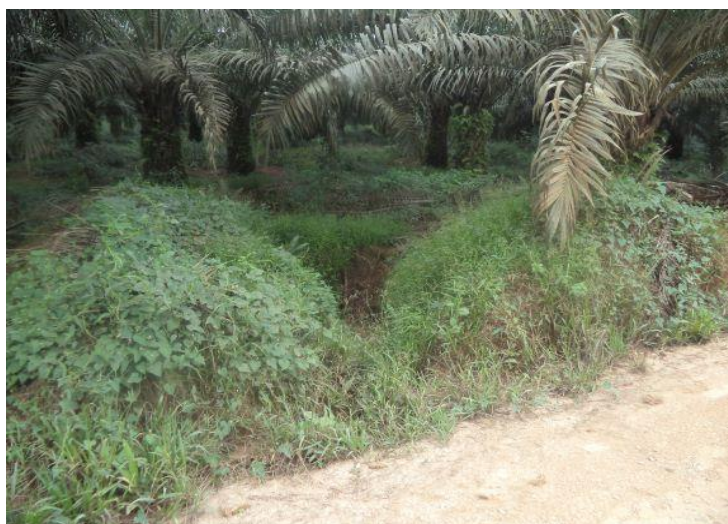
Plate 3.2: Sedimentation and/or Side Pit on Roads
