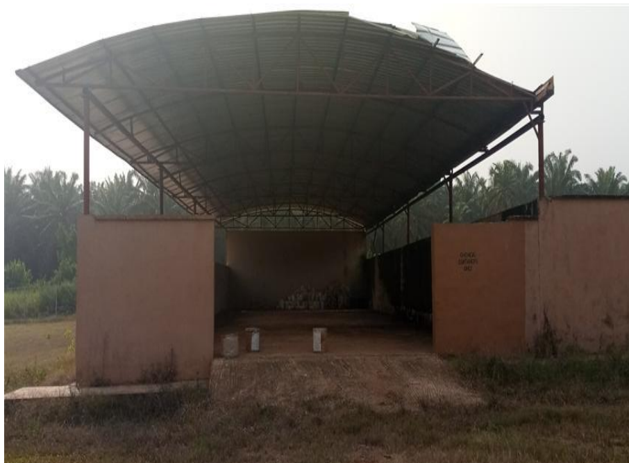
Plate 8: Empty Agrochemical Containers' Storage Compartment covered with roofing sheet to prevent run-off during rainfall
