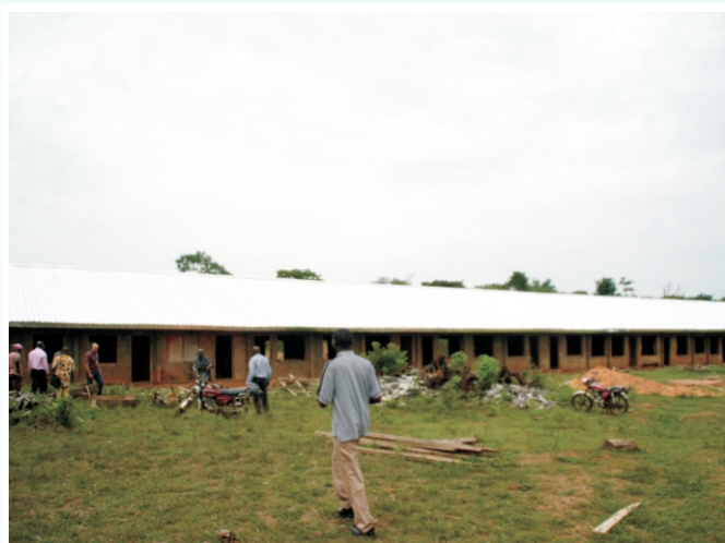
Inspection of Secondary Building at Oke, Ovia North East L.G
