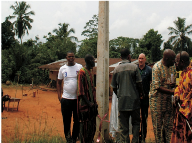
Electrification Work at Madagbayo
