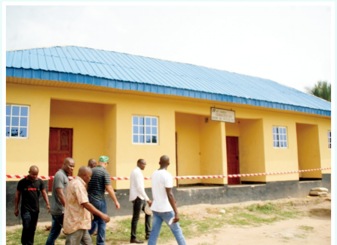
Teachers Quarters built by Okomu oil at Inikorogha, Ovia North West L.G
