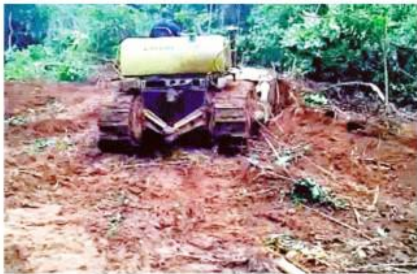
CONSTRUCTION OF OKOMU IJAW ROAD BY OKOMU OIL PALM CO. PLC
