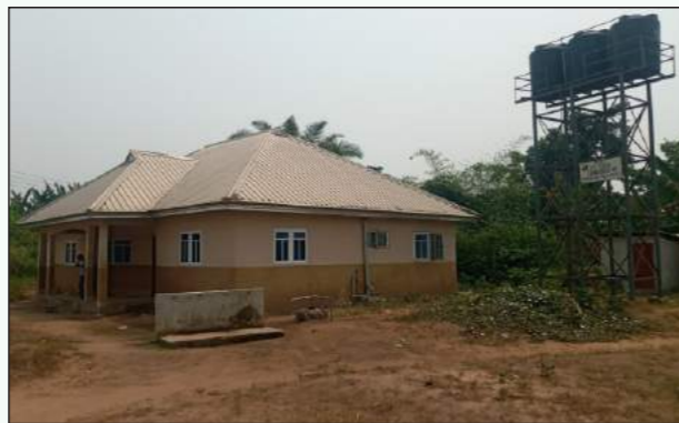
DOMESTIC BOREHOLE AT OFUNAMA COMMUNITY
