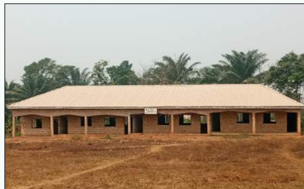
ONGOING BLOCK OF CLASSROOMS AT UHIERE COMMUNITY
