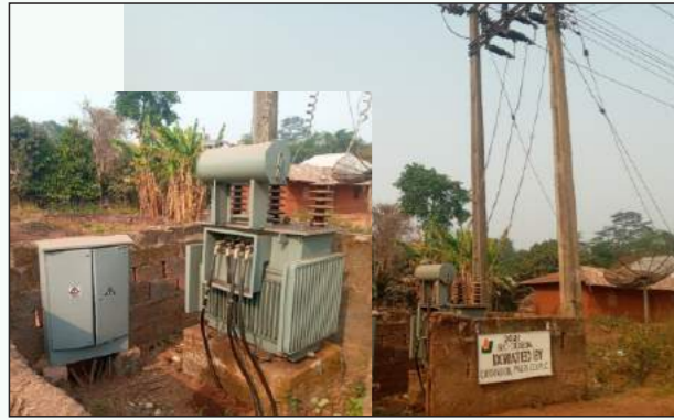
ELECTRICITY TRANSFORMER AT IRHUE COMMUNITY
