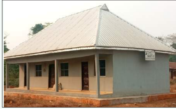
COMPLETED CORPERS' LODGE AT EKPAN COMMUNITY
