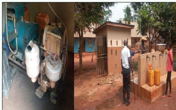
INDUSTRIAL BOREHOLE, GENERATOR HOUSE AND A GENERATING SET AT ODIGUETUE COMMUNITY
