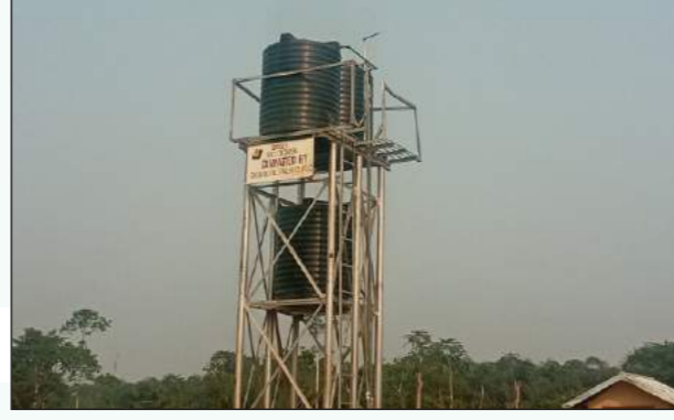
DOMESTIC BOREHOLE AT GBOLE-UBA COMMUNITY
