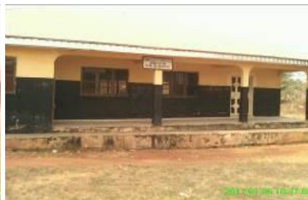
Plate 6: A block of classrooms built by OOPC at Secondary School, Udo
