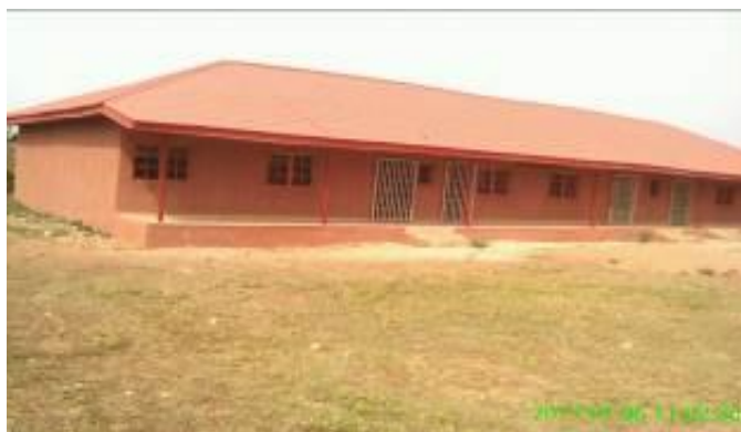
Plate 5: Renovated block of Emokpae Primary School, Udo
