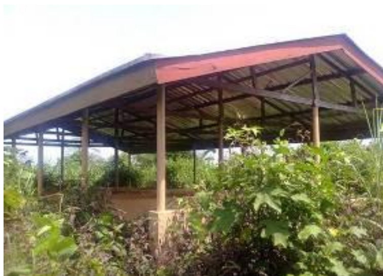
Plate 4: Open Market Stores Built by OOPC Covered with Weeds
