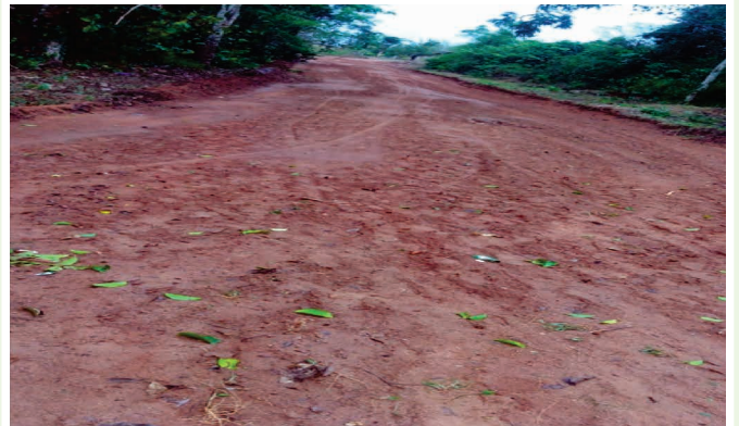
Grading of Road At Oke By Okomu
