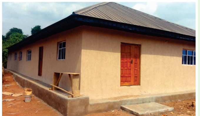
Community Hall At Irhue Built By Okomu
