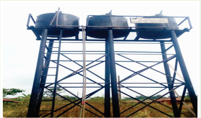
Borehole At Umokpe Constructed By Okomu
