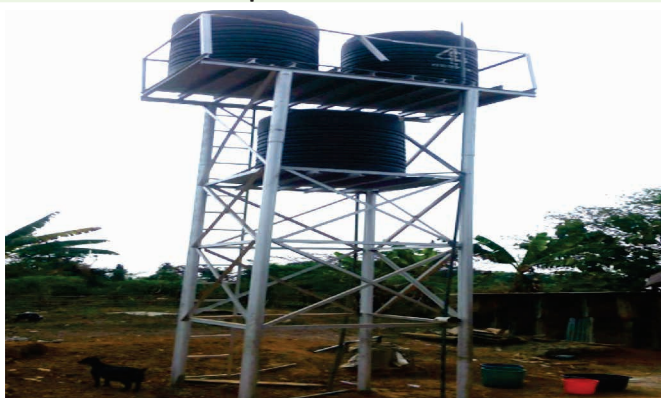
Borehole At Owan Donated By Okomu
