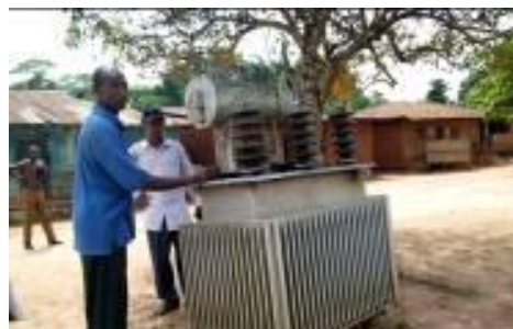
Transformer left uninstalled
