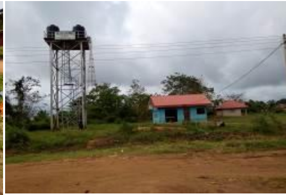
Plate 4-12; Odighi malfunction reticulated water scheme
